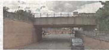
The footbridge over Kingsgate Road
